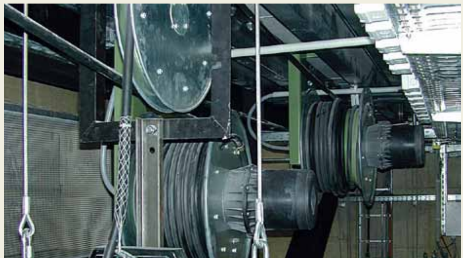
Cavotec Alfa spring driven reels are a common sight in theatre applications around the world.
