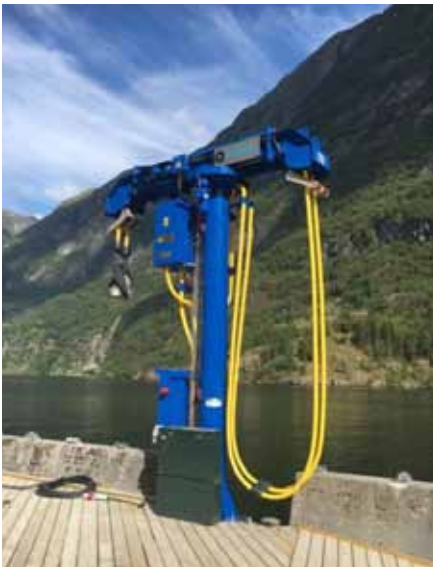
AMPDispenser installed at the Port of Gudvangen.
