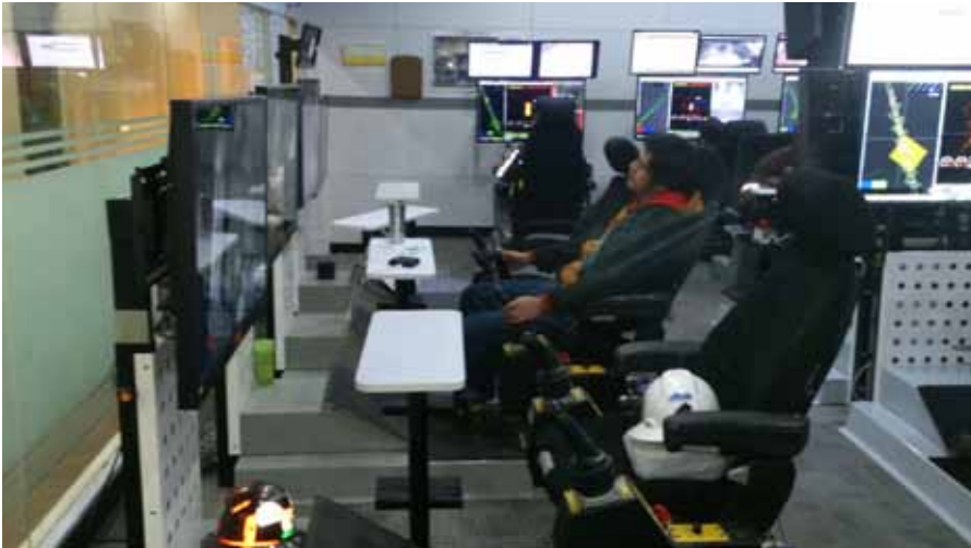
Control room, Freeport Mine
