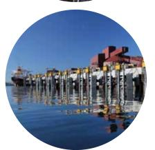
MM200C17 **Product:** Type: Front mounted Capacity:  $18 \times 200 \text{kN} = 360 \text{ tonnes}$ **Moorings:** 2-4 times a week Route: Global Various carriers up to 185,000 DWT **Vessel names:** LOA: up to 305m Operator: LKAB Owner: **LKAB** Since 2016 In operation:
