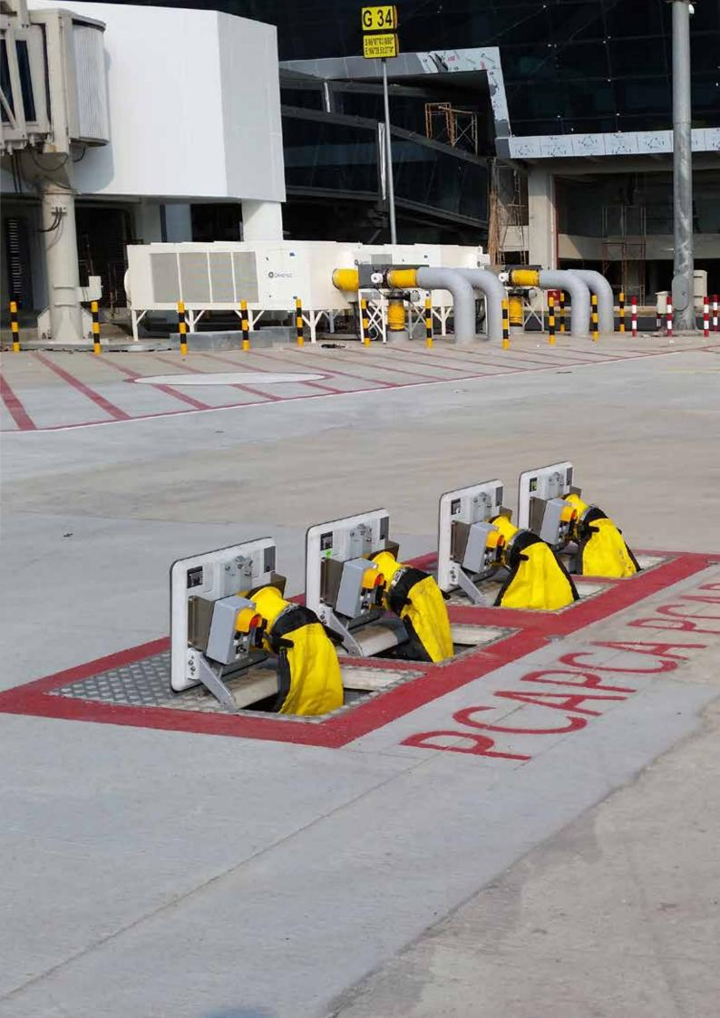
Cavotec manufactures a wide variety of Central and Point of Use PCA systems, including fixed, mobile, above-, in-ground, and subfreezing, all of which meet or exceed performance requirements.
