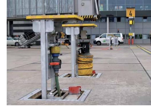
Cavotec's Wet Services System has been adopted by several airports. Its implementation has resulted in more efficient ground handling, reduced emissions and TAT.
